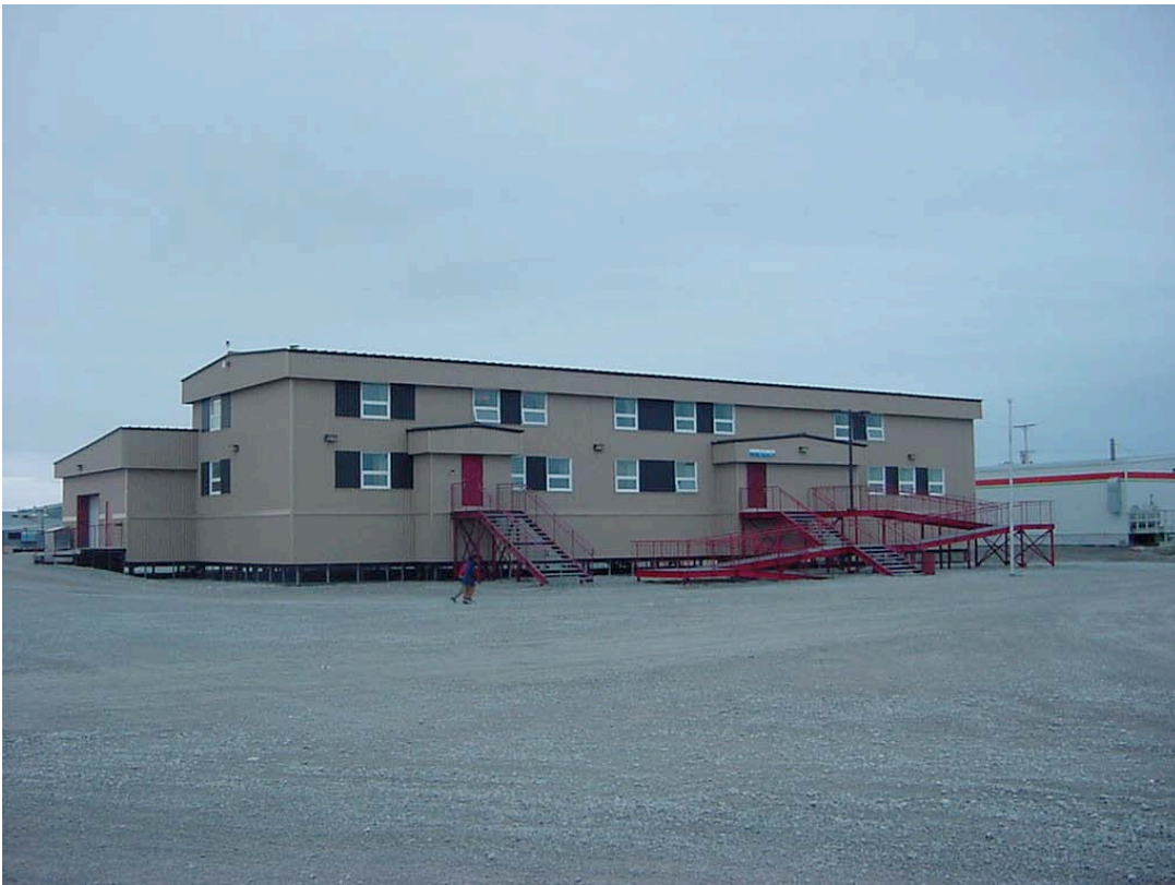
Hall Beach Health Centre, Anton North
