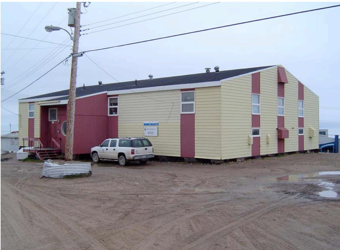
Pond Inlet Health Centre, Anton North
